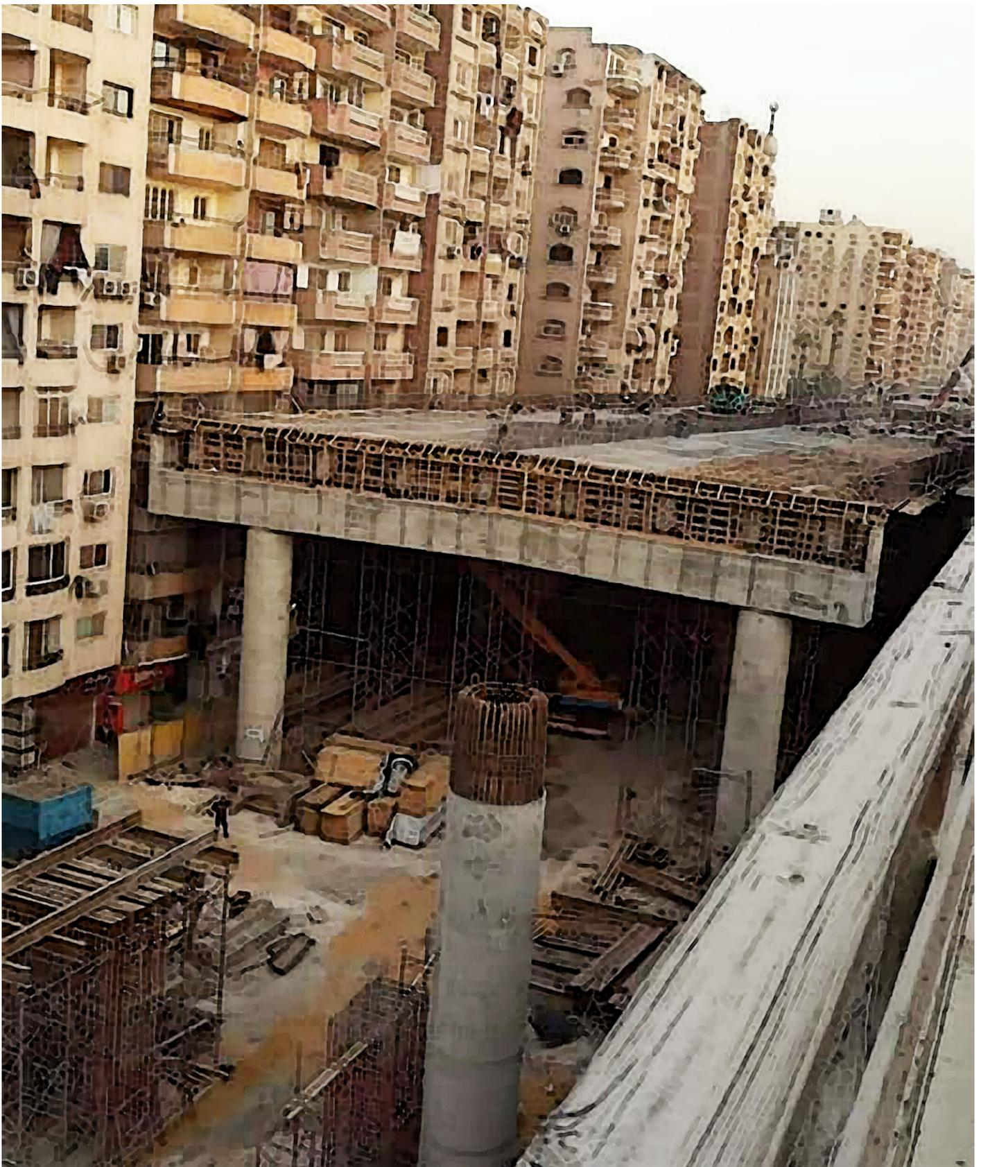
Figure 1: Where urban transport systems and residential functions meet. The picture shows the construction of the Teraet Al-Zomor Bridge in Cairo. Its edges are within arm's reach of people's balconies and it overshadows at least four storeys. Image credit: Mostnir Shady Ahmed (2020), <https://www.facebook.com/mostnir/posts/10221856461623192> (Accessed on 26 Feb 2021). Printed with permission.
