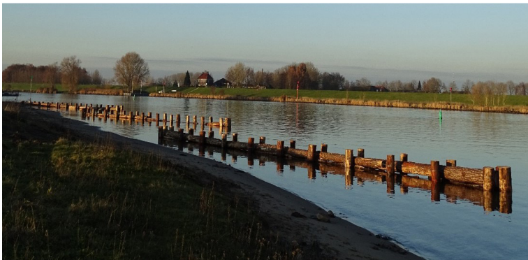
8-30. Wooden screens to prevent bank erosion. © BAM / Van den Herik
