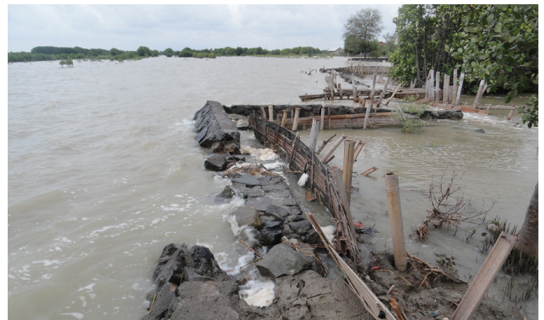
4-48. Failing sea wall along the Demak coast. © Wetlands International
