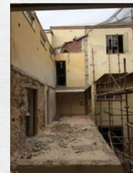
BEFORE: Floor joists to be supported by the steel portal frame. Photographs: CCT
